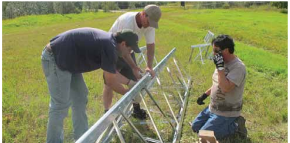
Crews installing a wireless transmission tower in Doig River.
